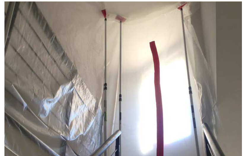
Quick Props provides an instant barrier between the working environment and surrounding areas
