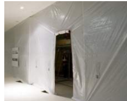
Self-adhesive zippers easily adhere to the screening material.
